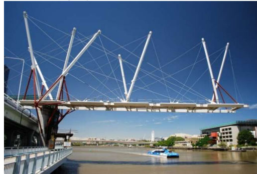
Σχ. 5: Brisbane Bridge, Australia – Tensegrity bridge
